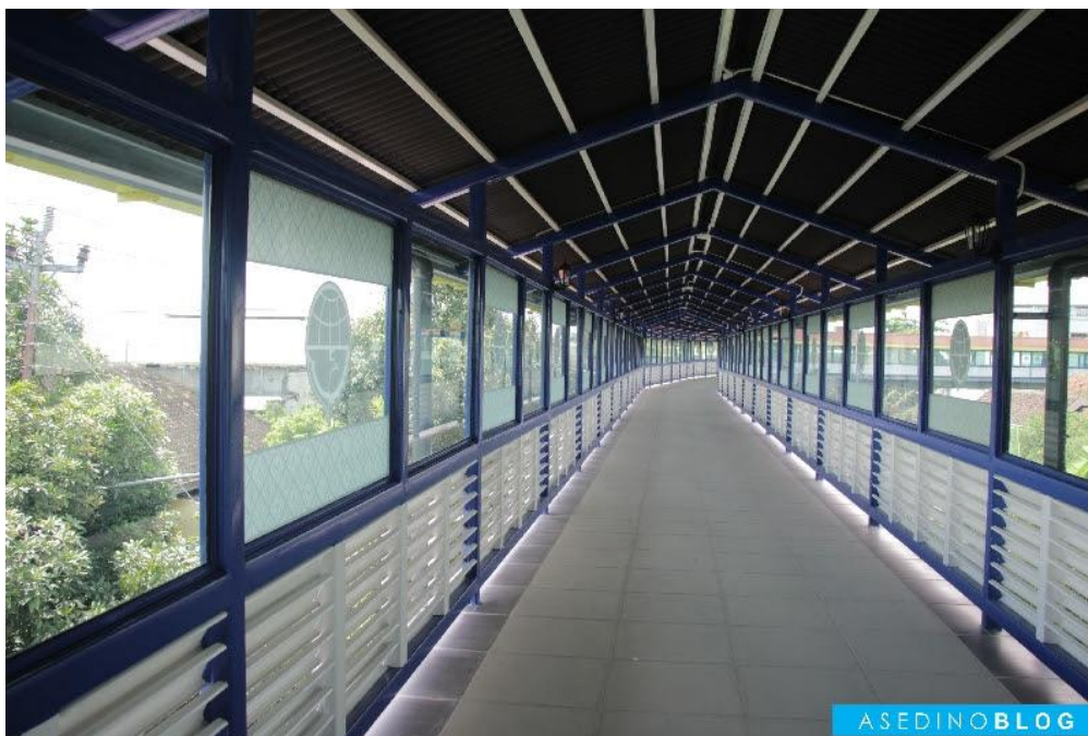
Gambar 4 Skybridge stasiun Solobalapan ke terminal Tirtonadi (asedino.wordpress.com, 2017)
