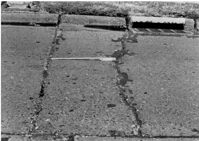
FIG. X2.35 Low-Severity Punchout
