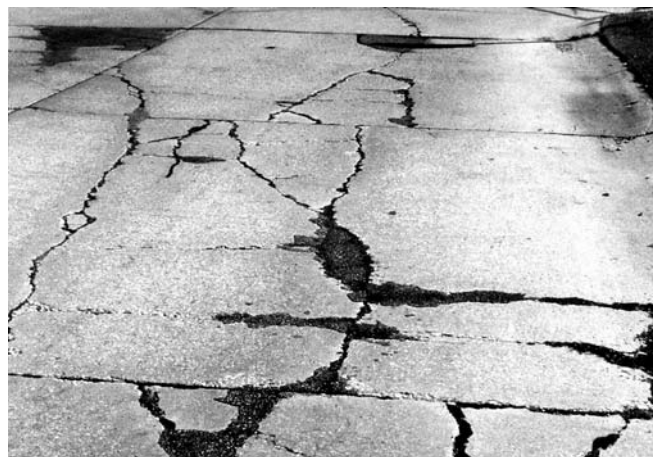
FIG. X2.9 High-Severity Divided Slab
