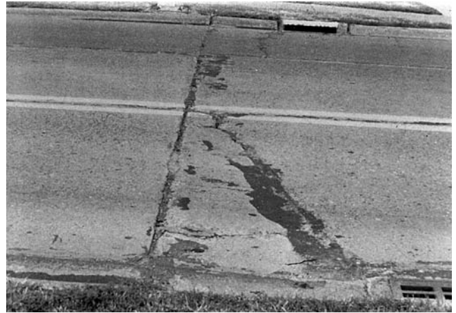
FIG. X2.36 Medium-Severity Punchout
