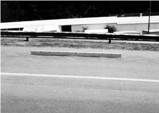
FIG. X1.14 Medium-Severity Corrugation
