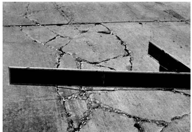
FIG. X2.37 High-Severity Punchout
