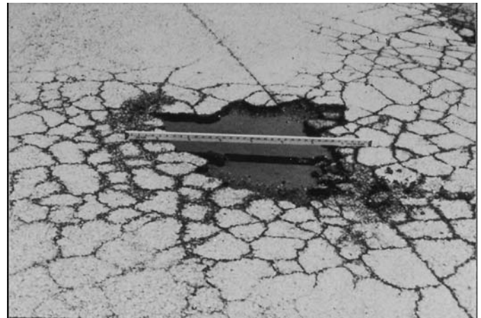
FIG. X1.37 High-Severity Pothole
