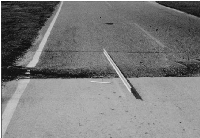
FIG. X1.46 High-Severity Shoving
