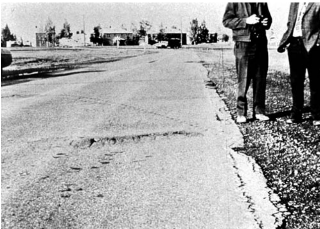
FIG. X1.11 Medium-Severity Bumps and Sags
