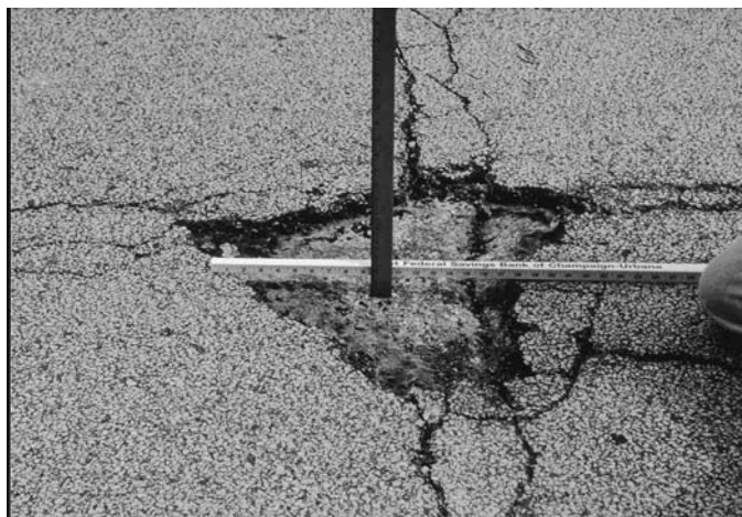
FIG. X1.36 Medium-Severity Pothole
