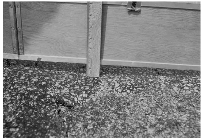
FIG. X1.43 High-Severity Rutting
