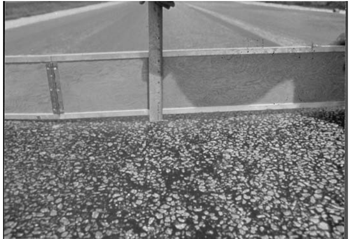
FIG. X1.42 Medium-Severity Rutting
