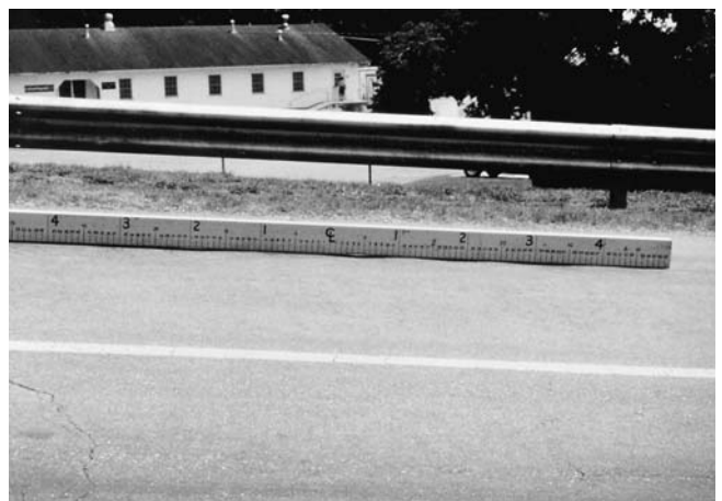
FIG. X1.13 Low-Severity Corrugation
