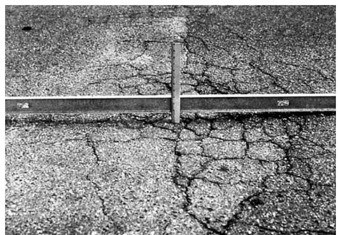
FIG. X1.18 High-Severity Depression
