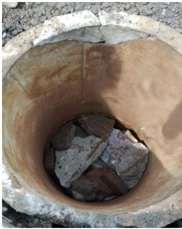
Gambar 6. Proses Pengisian Batu Pecah kedalam Sumur Resapan
