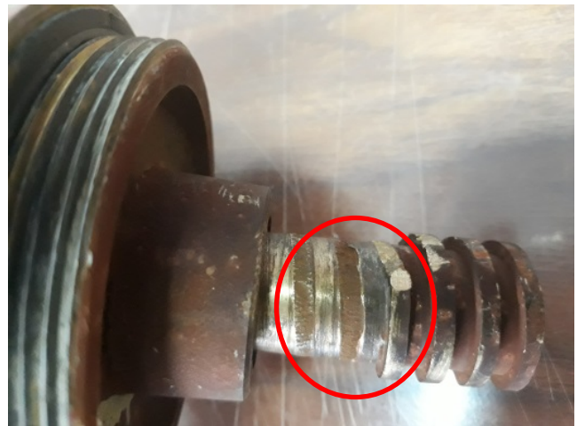
Figure 5. Fracture at Thread of Stem Valve
