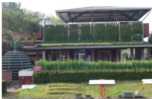
Figure 5. Research Center for Environmental Science and Technology Rainwater Recycling System
