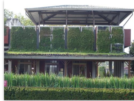
Figure 10a. Plant wall cultivated with treated wastewater
