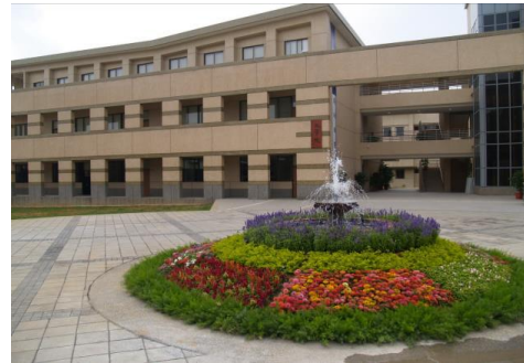
Figure 4. College of Engineering Recycled Rainwater Watering System
