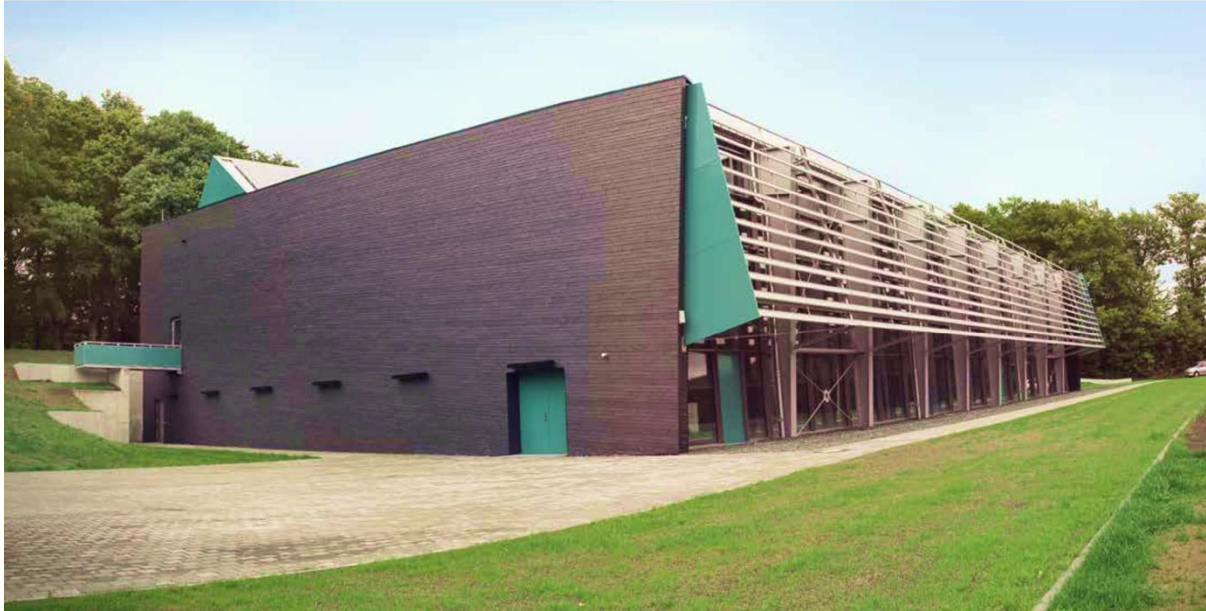
Figure 7. Multifunctional Gymnasium with smart shadowing and air conditioning [4]
