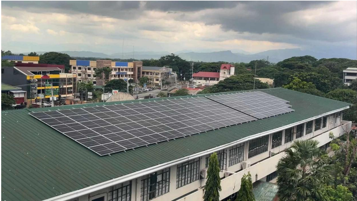
Figure 1. The installation of solar PV system on SBE building
