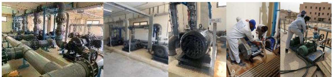
Figure 12. Pumps for pumping treated water.
