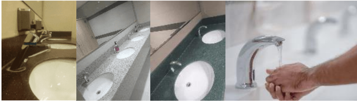
Figure 17. Automated hand washing taps in Qassim University.
