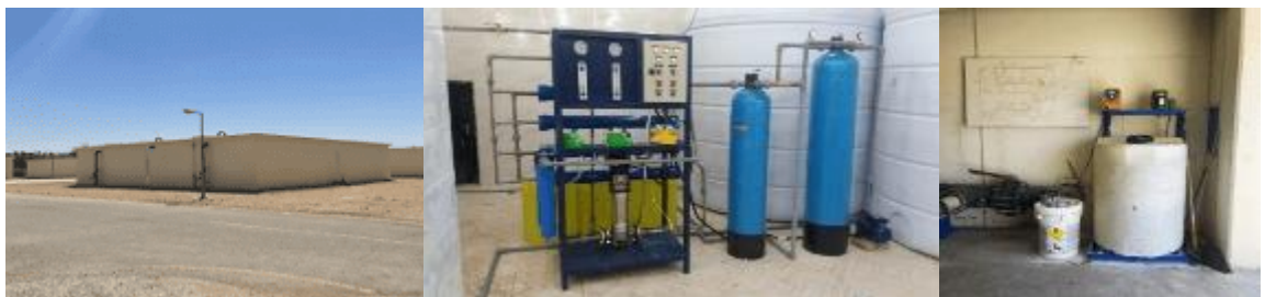
Figure 11. Irrigation water tanks and Sterilization unit.
