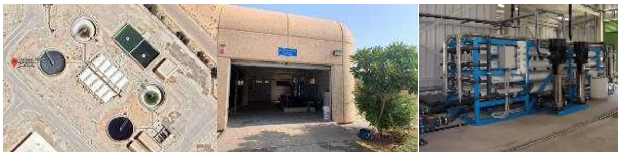
Figure 5. Water Recycling Station in Qassim University
