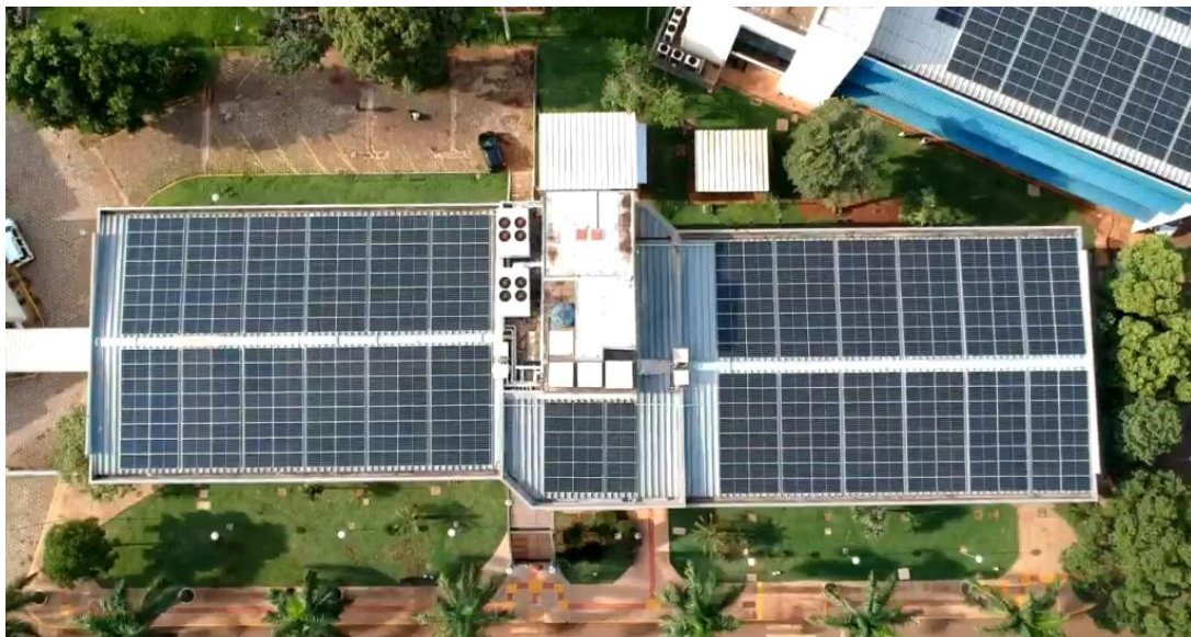
Figure 2. Photovoltaic Solar Panels on UFMS Buildings
