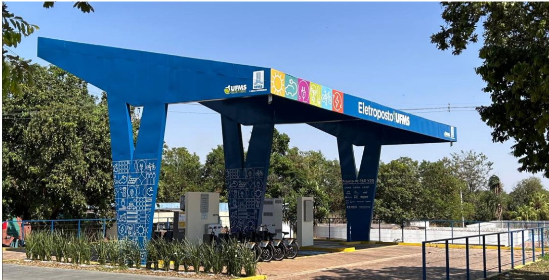
Figure 3. UFMS Electrostation: Recharging Electric Cars and Bicycles
