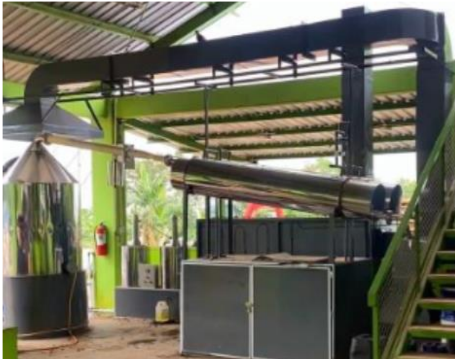
Figure 7. Pyrolysis condition in TPST Undip
