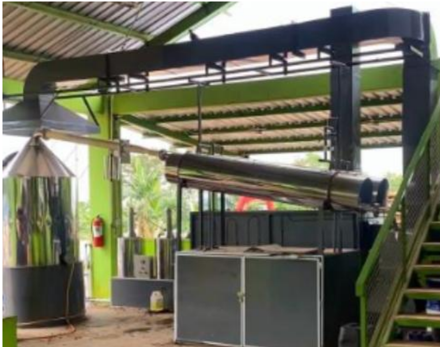
Figure 7. Pyrolysis condition in TPST Undip
