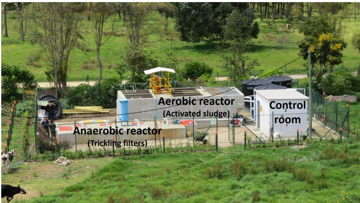
Figure 3. Wastewater Treatment Plant (main WWTP) in 2014
