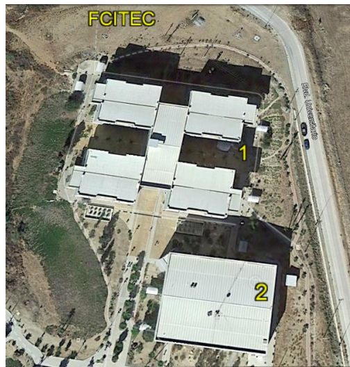
Figure 19.- Rainwater collection potential on roofs, building 1 (“Prisma”) and building 2 (Administrative) of FCITEC. Source: Google Earth, 2023.
