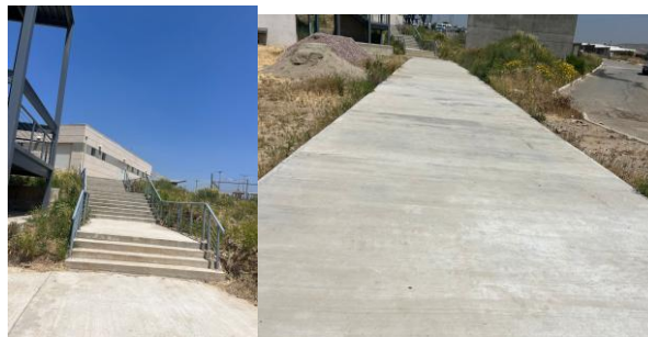
Figure 4. Access from parking lot 3 to the bus stop
