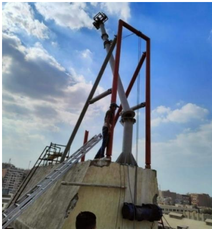
Figure 3. The WT tower during erection tests
