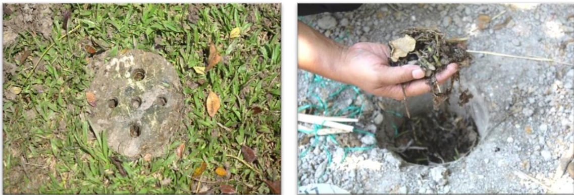
Figure 2. Biopore infiltration hole for water
