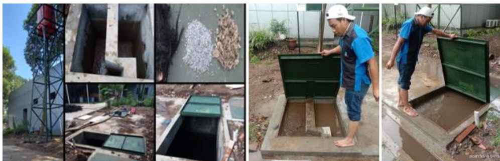
Figure 5. Implementation of rainwater harvesting construction in the area of Alor Building
