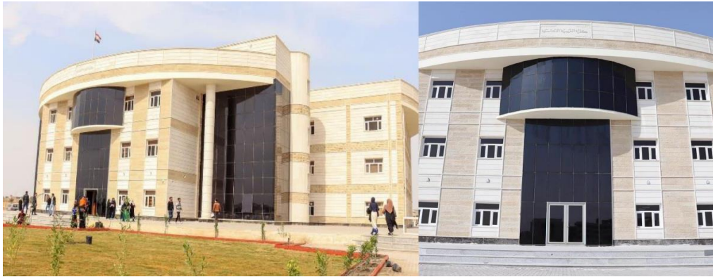
Figure 3. Shows the Double-glazed Technique in on of MU Campus Buildings Façade
