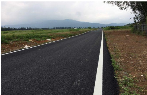
Figure 7a. Water permeable asphalt roads
