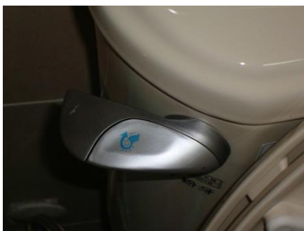
Figure 8a. Dual flush toilettes
