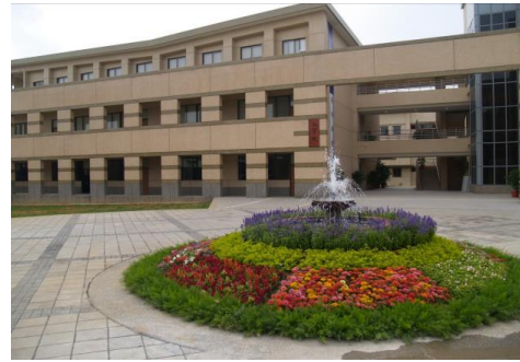
Figure 4. College of Engineering Recycled Rainwater Watering System
