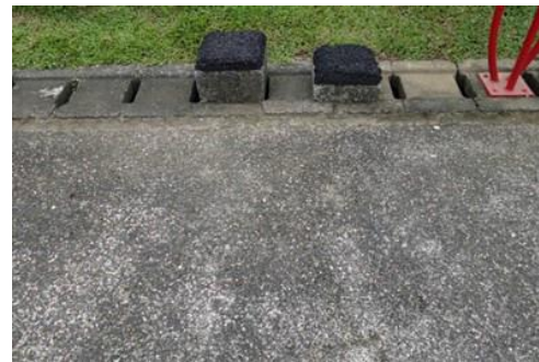
Figure 7b. Water permeable walkways and parking lots
