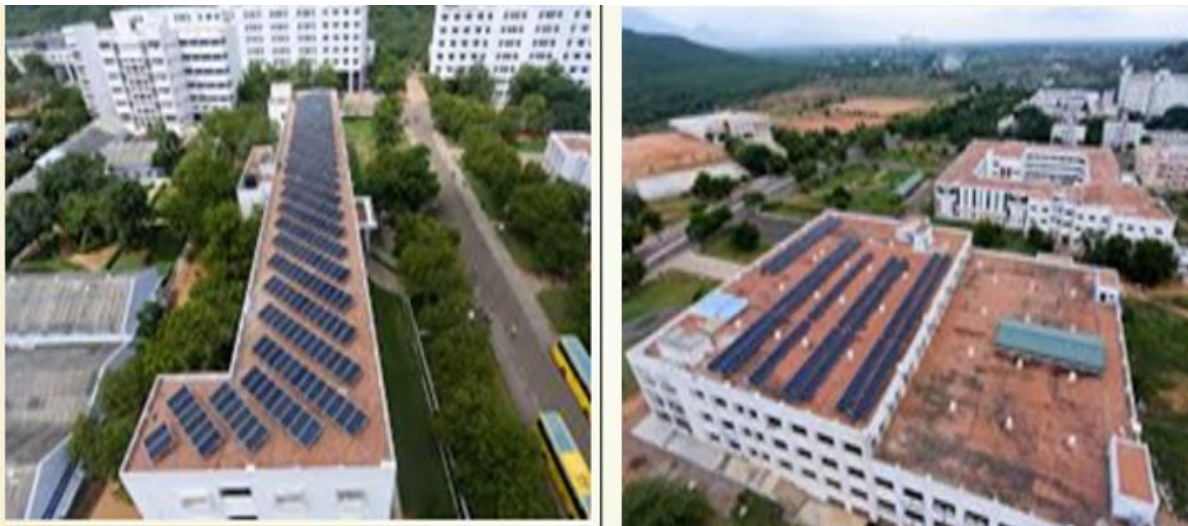
Figure. 1 Some of the solar panels installed on the campus
