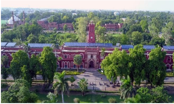
Figure 7. Rooftop Solar PV plant around the iconic Victoria Gate of AMU
