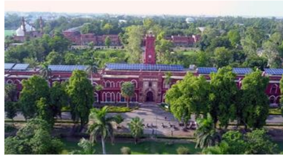
Figure 2. Rooftop Solar PV plant around the iconic Victoria Gate of AMU
