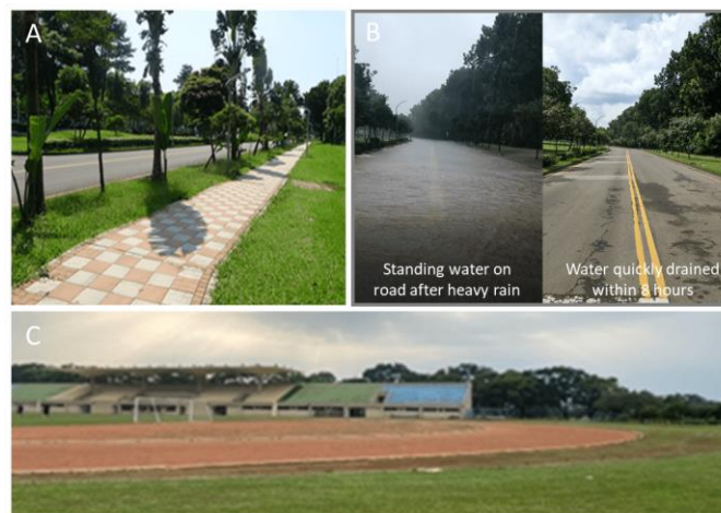
Figure 1. A. Permeable pedestrian pavement, B. The permeable asphalt pavement help standing water drain quickly after a heavy rain. C. Red clay surface of the race track.
