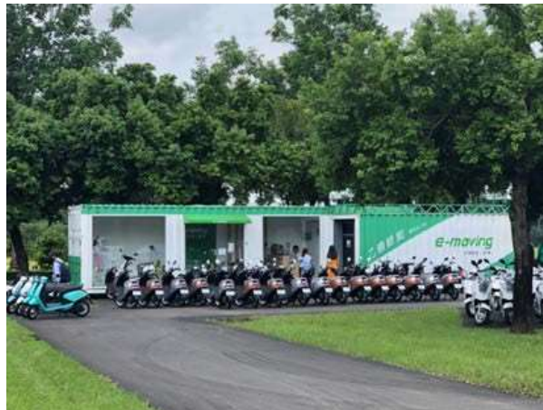
Figure 5. Electric bicycle/motorcycle charging station
