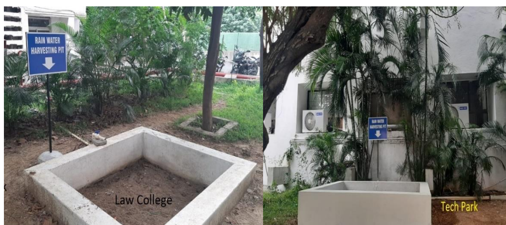
Figure 5. Rain Water Harvest Pit at SRM
