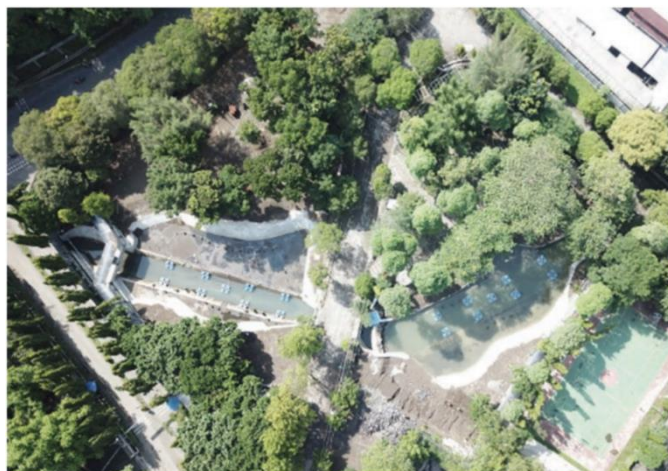
Figure 7. Storm-water drainage system in the Faculty of Engineering UGM
