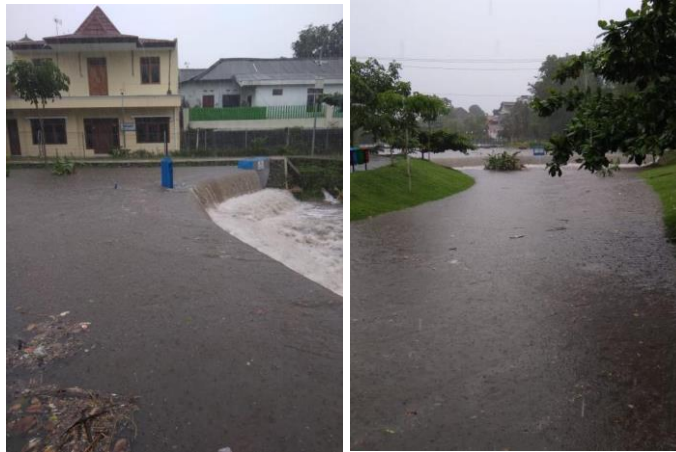
Figure 6. Storm-water drainage system in Wisdom Park UGM
