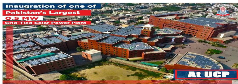
Figure 2. Inauguration of 0.5 MW Grid-Tied Solar Power Plant at UCP, Lahore on all rooftop structures
