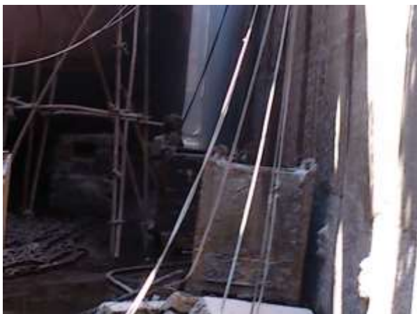
Gambar 6. Proses Sandblasting
