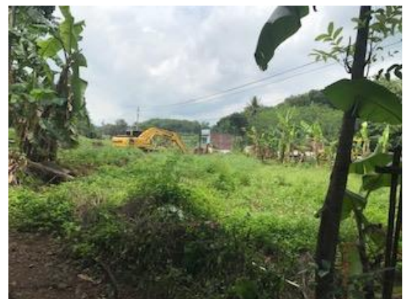
Figure 2. Rencana Lokasi Rest Area
