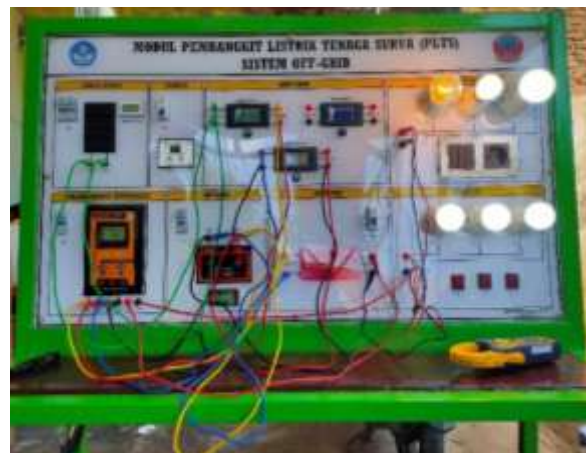
Gambar 5. Pengujian Solar Charge Controller
