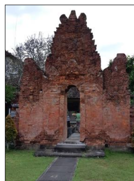
Figure 3. Main gate of Kesiman Palace made of brick stone. Craftmanship for making brick stone construction has been rare found today
