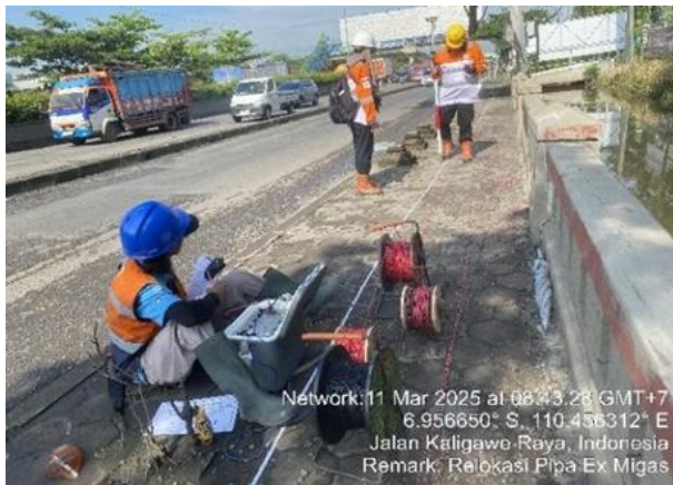
Gambar 3. Pekerjaan soil resistivity test
