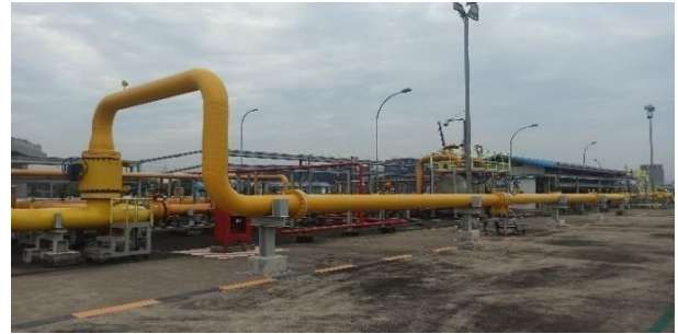
Gambar 9. Bypass slug catcher after konstruksi
