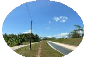
Jaringan fiber optic (313 km)
