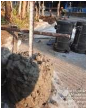
Gambar 6. Slump test beton
