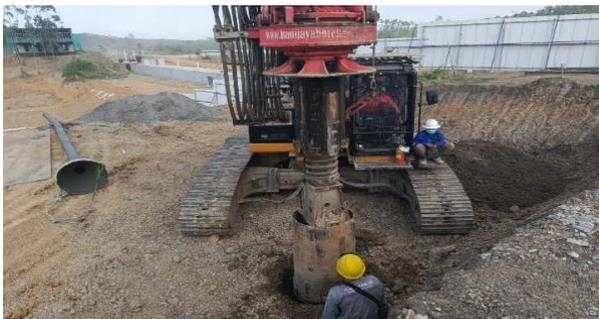
**Gambar 5.** *Rock auger/core barrel*
