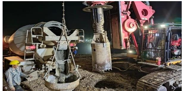
Gambar 8. Pengecoran *bored pile*
