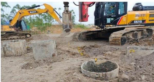
**Gambar 6.** *Casing pipe*
