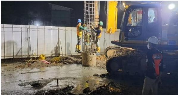
Gambar 7. Instalasi *steel cage*
