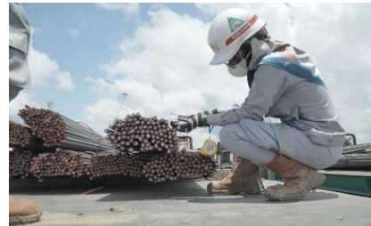
Gambar 4. Pengecekan incoming baja tulangan
