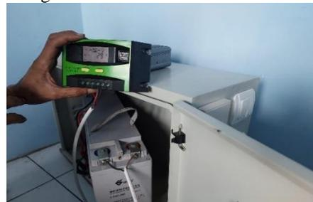
**Gambar 5.** Pemasangan solar charge controller
