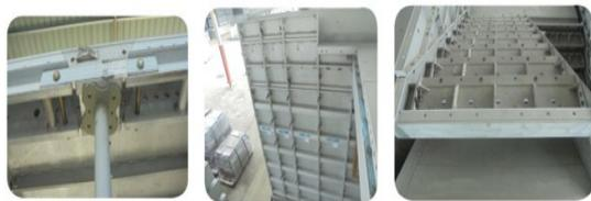
Gambar 5. Fix Shoring, Bekisting Shearwall dan Tangga
