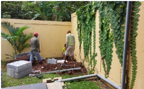
Gambar 8. Proses pengerjaan Rain Water Harvesting .
