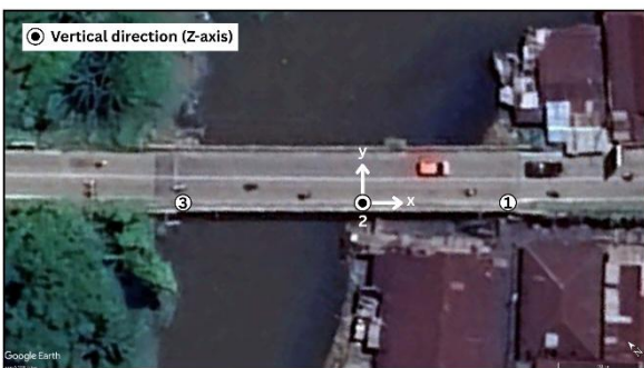
Fig. 4: Measurement points on Jembatan Jalan Gelatik, Samarinda (Source: Google Earth)
