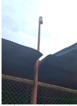
Fig. 2 : Installation of SQM in the zenith direction
