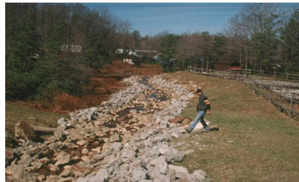
Gambar 2. Ilustrasi *Open Limestone Channel* (Skousen *et al*, 2016)
