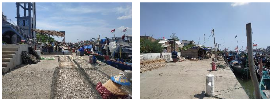
Figure 3.2. Dock's Condition (Author, 2020).
