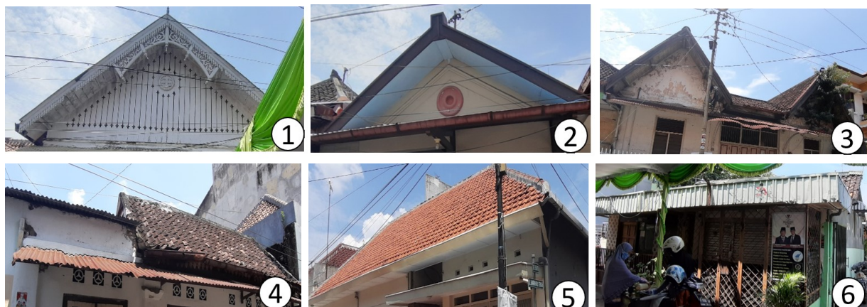
Figure 3.2. Typology of Building Roofs on Bangunharjo street (author, 2019)
