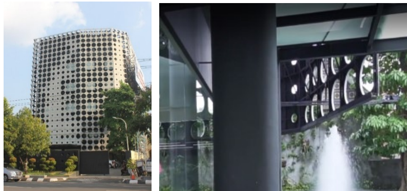
Figure 3.1. GRC Facade of Wisma Anugerah (authors, 2019)
