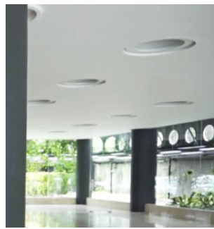
Figure 3.3. GRC Installed as Ceiling (authors, 2019)
