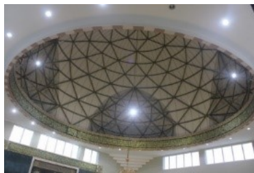
Figure 3.15. Dome Interior (authors, 2019)
