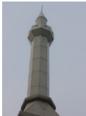
Figure 3.16. Cladding of GRC Tower (authors, 2019)
