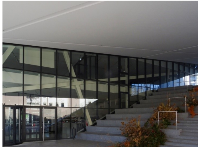
Figure. 3.6. The steps and the entrance (author's photo, 2018)
