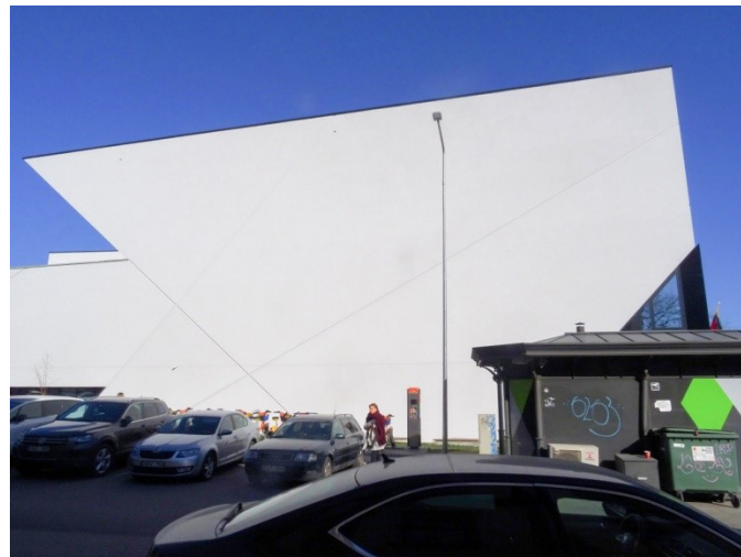
Figure 3.2 Side façade as blind curtain wall (author's photo 2018)
