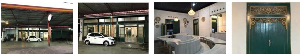
Figure 1.5. Hidden authentic joglo roof by additional iron roof (a), Additional glass material at front door (b), Modern concept interior (c), Repainted authentic door ornament (d) (Author, 2023)
