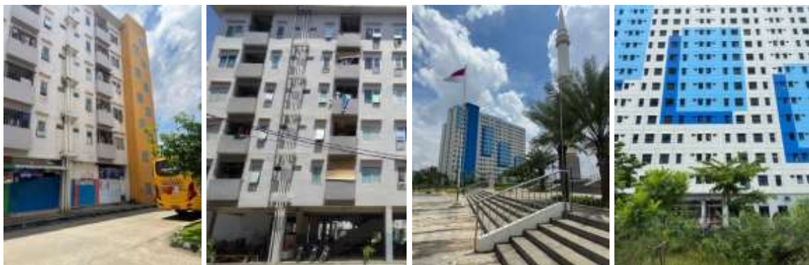
Figure 2.2. Rusunawa Pesakih. (The first two pictures from the left are middle-rise; the rest are high-rise.) (Private documentation, 2023)
