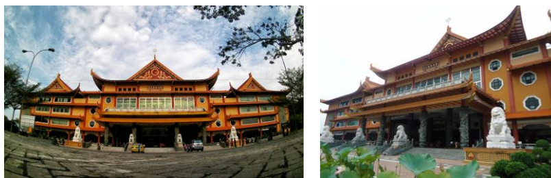
Figure 1. The front view of Great Maitreya Temple (Source: Phinemo, 2017 and Indozone, 2020)
