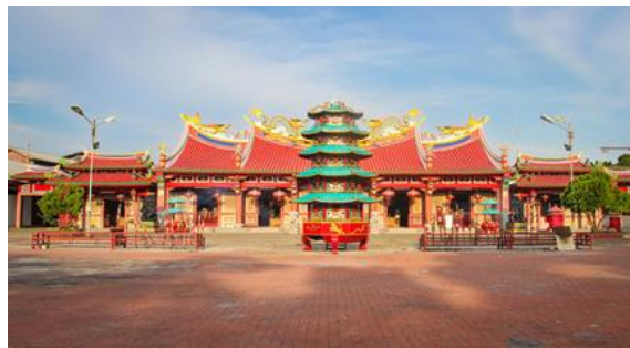
Figure 3. The front view of East Mountain Temple (Source: Jurnal Asia, 2014)
