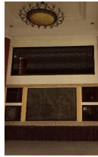
Figure 8. Openings, windows, and vents on wall (Source: Personal Documentation, 2021)
