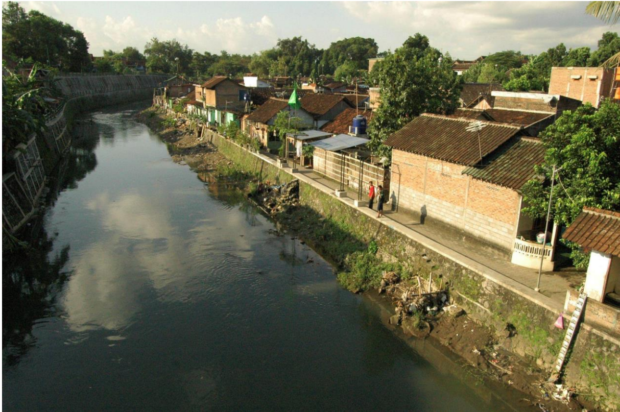
Figure 3.2. The condition of the embankment and LIC settlements in Kampung Suranatan (Author Observation, 2022)
