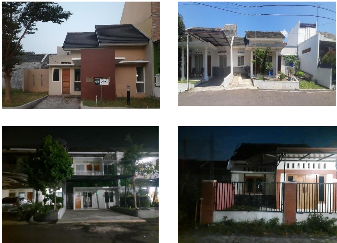
Figure 3.9. Façade of Residential Unit Source: Author survey, September 2021
